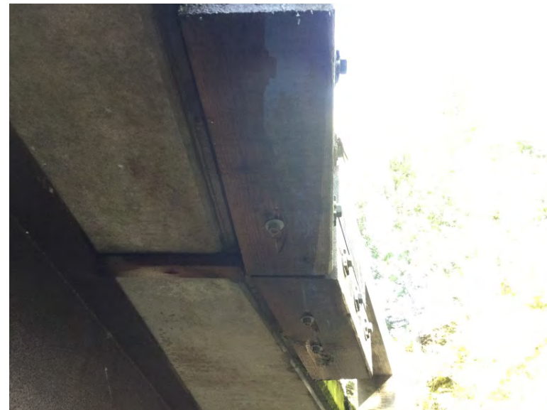
Missed rail bolt and only small washers used
