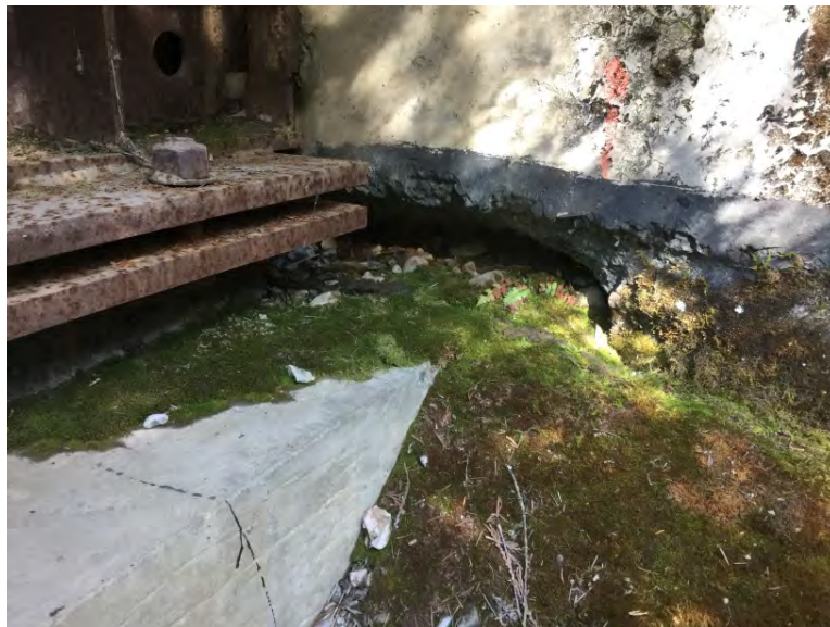
Ballast wall appears to have been cut to fit over CIP at upstream right bank
