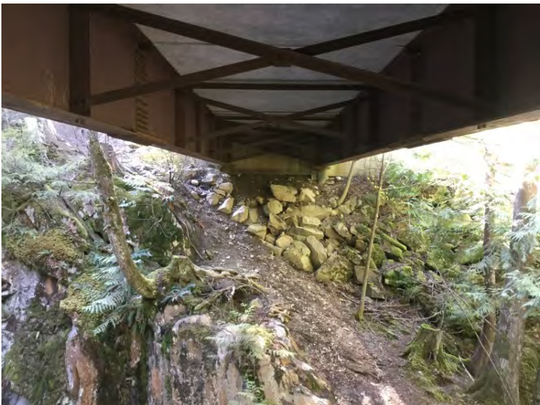
Left Bank Abutment when facing downstream
